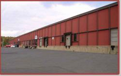
MAIN FEATURES -Clear Height: 16ft. Above finished floor to underside of structural steel -Exterior: Insulated wall panel -Glass wall system at offices
